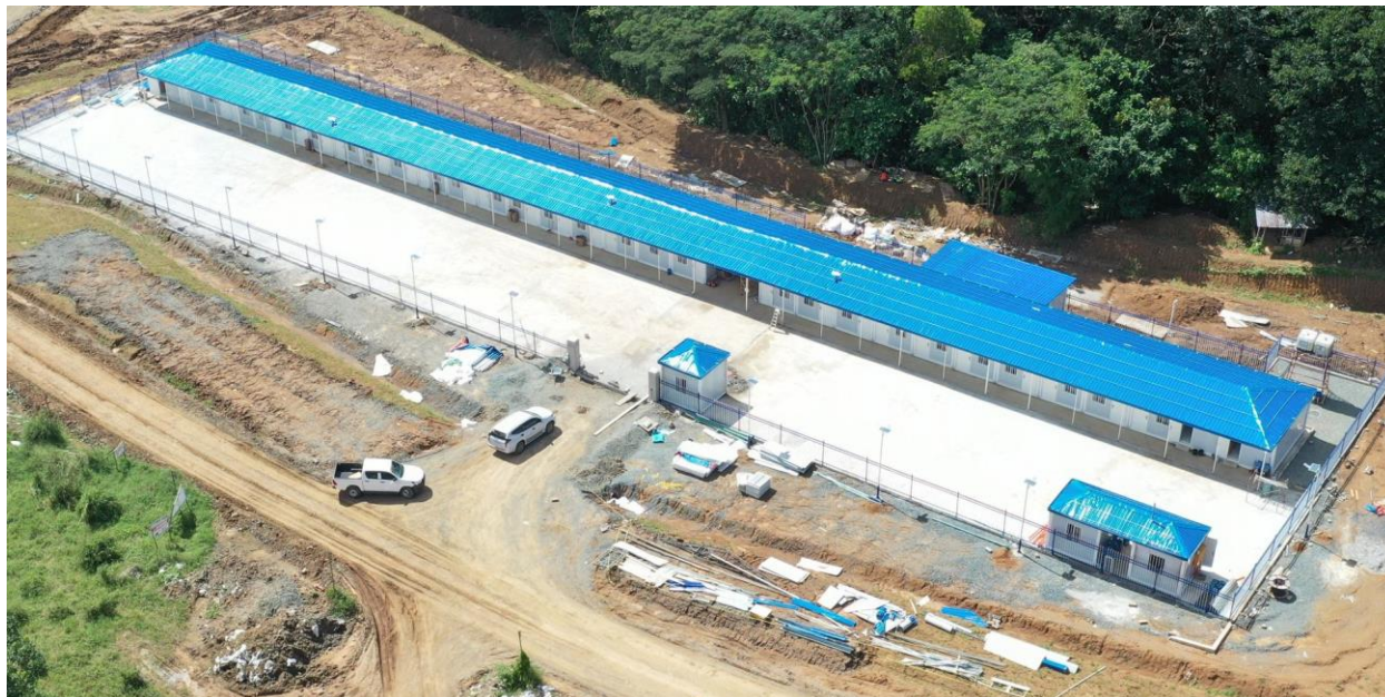
Newly built temfacil (temporary facility) serving as the project site office for the construction of the Tanay Wind Power Project
