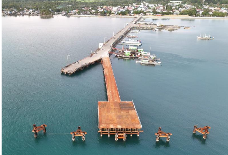
Temporary jetty completed for Alternergy's 64 MW Alabat Wind Project on Alabat island, Quezon Province
