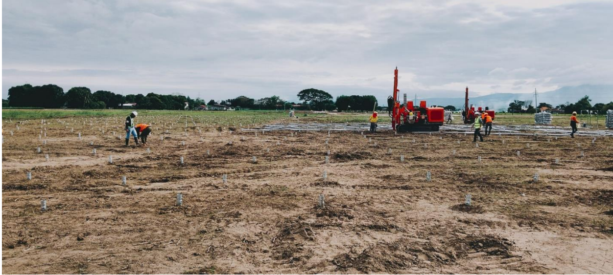
Ongoing construction of Alternergy's 28 MWp Balsik Solar Power Project in Hermosa, Bataan
