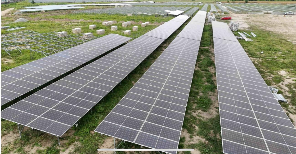
Ongoing construction of Alternergy's 28 MWp Balsik Solar Power Project in Hermosa, Bataan
