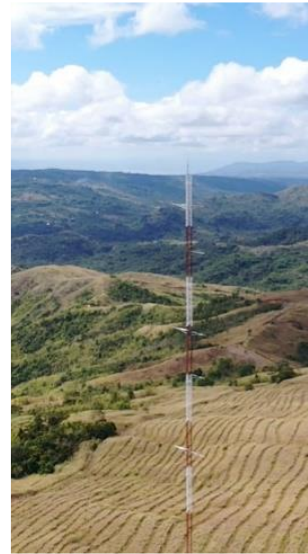
Tanay Wind Power Project Tanay, Rizal
