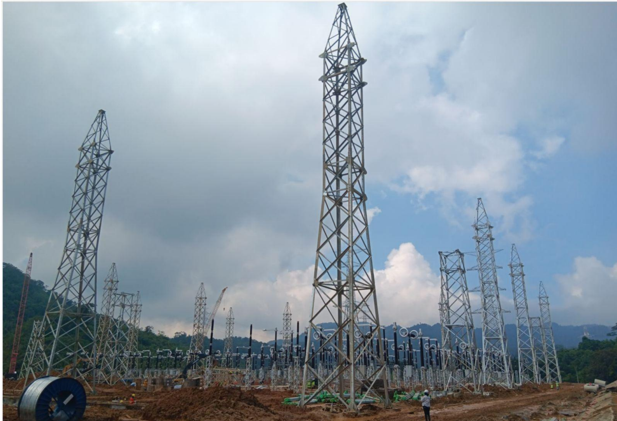
Construction of the Alternergy Tanay Wind Power Project Switchyard near completion
